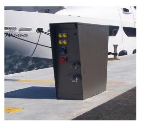
Figure 2.31 Typical service bollard
