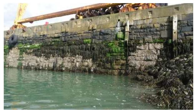
Figure 16.4 View along façade of stone-built quay (ADCO 03) in 2017 before it was buried in the development of Berth 2. The stone work was constructed above the 100-ton blocks that served as the foundation element to the quay.
